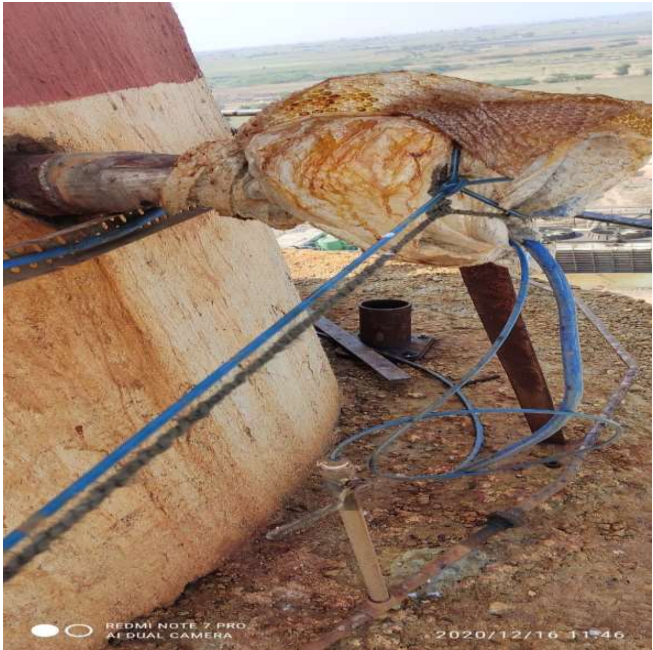
Stack monitoring equipment
