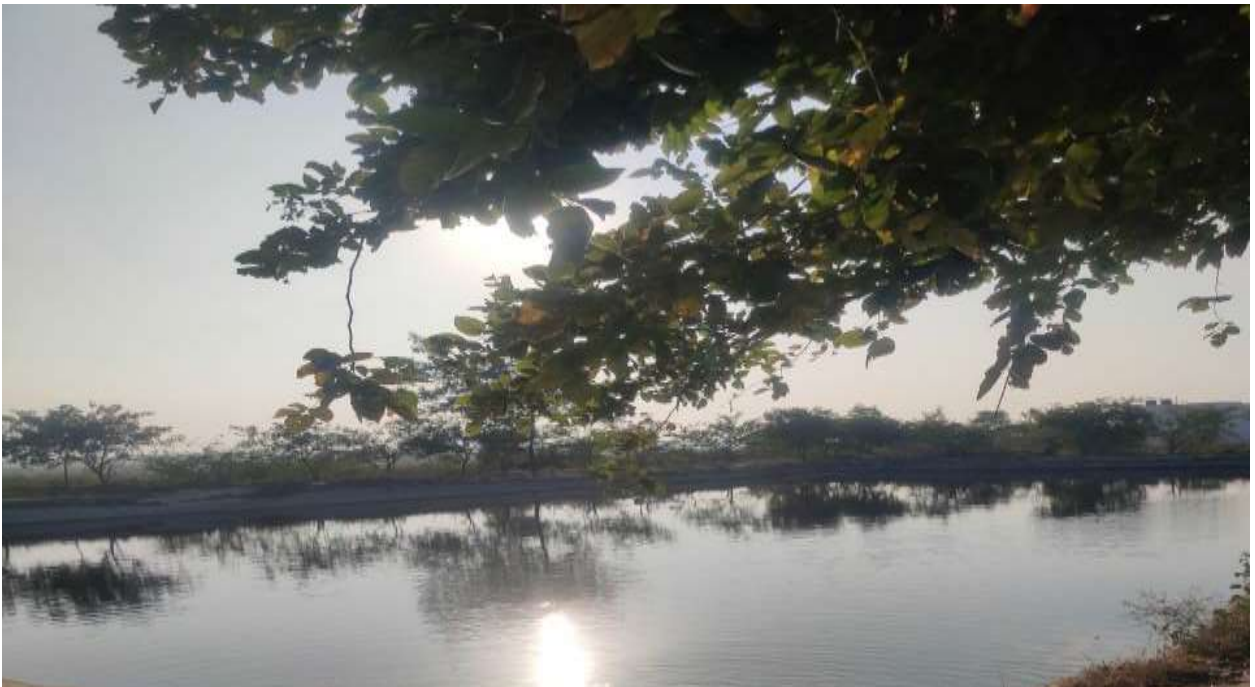
Rain water storage tank
