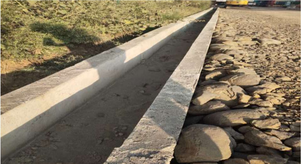
Storm water drainage
